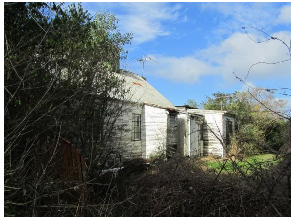
THE REAR OF THE COTTAGE
