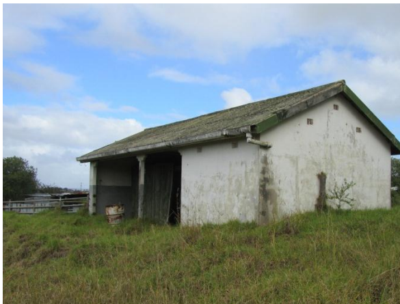
VIEW TO THE FORMER DAIRY BUILDING SHOWING THE PRINCIPAL NORTH EASTERN ELEVATION
