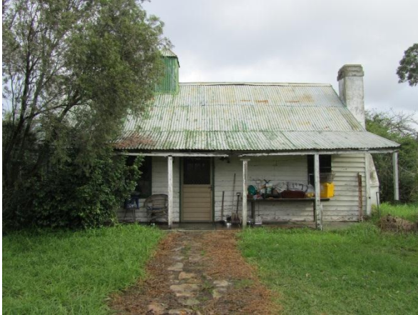
VIEW OF THE PRINCIPAL NORTH EASTERN ELEVATION
