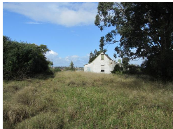
VIEW TO THE FORMER STABLES BUILDING FROM THE VARROVILLE HOMESTEAD BOUNDARY
