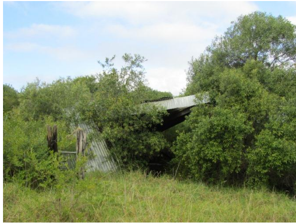
DERELICT CORRUGATED IRON STRUCTURE IN THE VICINITY OF THE DAIRY
