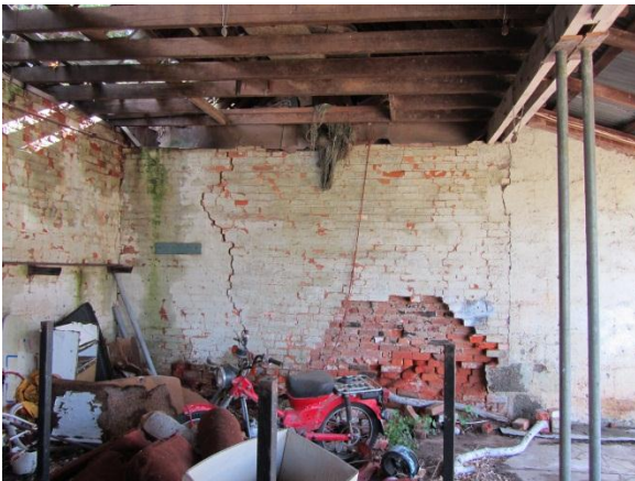
INTERIOR OF THE FORMER STABLES – VIEW NORTH
