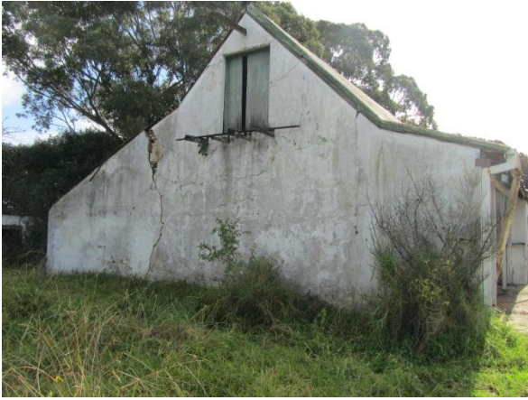
SOUTH EASTERN ELEVATION SHOWING THE OPENING INTO THE ROOF
