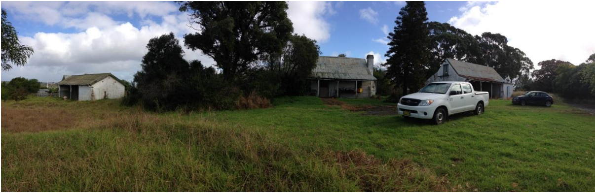
VIEW OF THE FORMER FARM BUILDING, COTTAGE AND STABLES BUILDING (FROM LEFT TO RIGHT)
