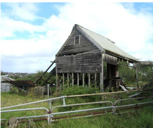
THE GABLED TIMBER WEATHERBOARD FORMER DAIRY BUILDING
