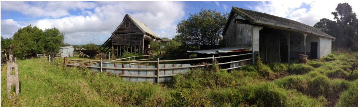
FORMER DAIRY BUILDINGS
