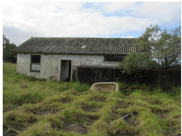
VIEW TO THE REAR OF THE FORMER DAIRY BUILDING INCLUDING ATTACHED ANIMAL STALLS
