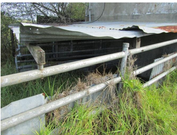
CONTEMPORARY FENCING ATTACHED TO THE MASONRY DAIRY BUILDING
